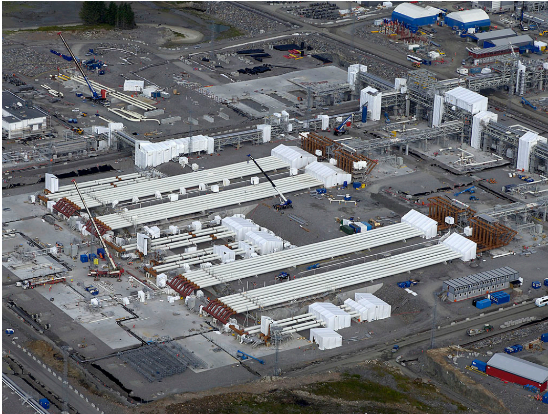
Ormen Lange Onshore facility
