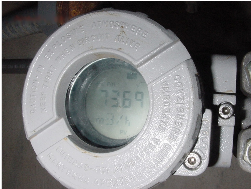
Figure 3. HART-based smart instrument indicating flow rate (PV measured in \text{m}^3/\text{hr} )
