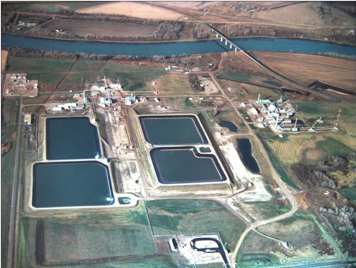
BP Canada Energy Plant - Fort Saskatchewan
